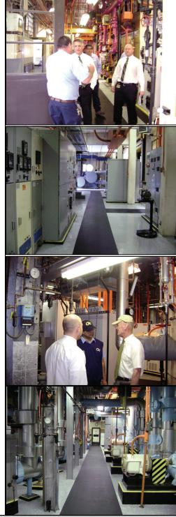
**1995** installed #1 @ 1000 tons (Carrier), in 1996 installed # 2 @ 1000 tons (Carrier), 1997 Removed original wood cooling tower, installed new 24,000gpm 8000ton Induced Draft Counter Flow.
