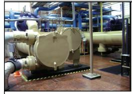
Was built in early 1900's, the Holland Plant is responsible for heating and cooling many of the buildings on Georgia Tech's campus. Chilled water and steam are produced at the Holland Plant and then sent out to the buildings on campus through a network of pipes and valves. The Holland
